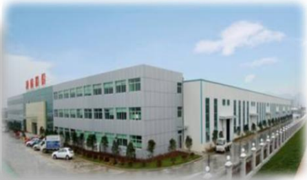
Domestic pump factory
